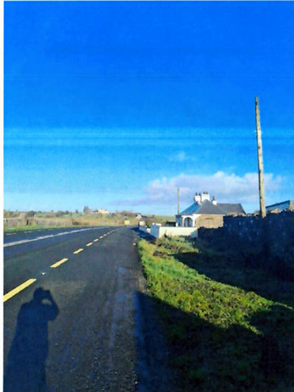
Photo I – The 110KVA line from Clough to Cloone in Tuam.
